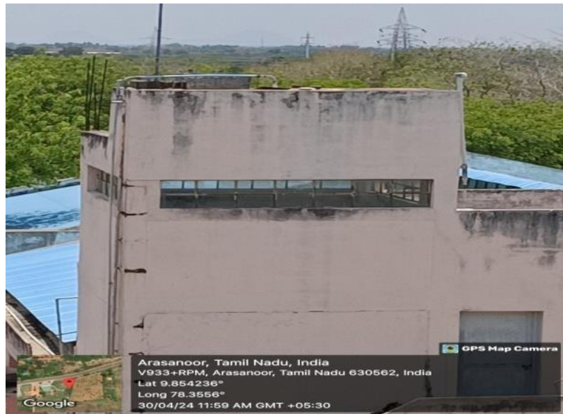
WATER STORAGE TANKS
