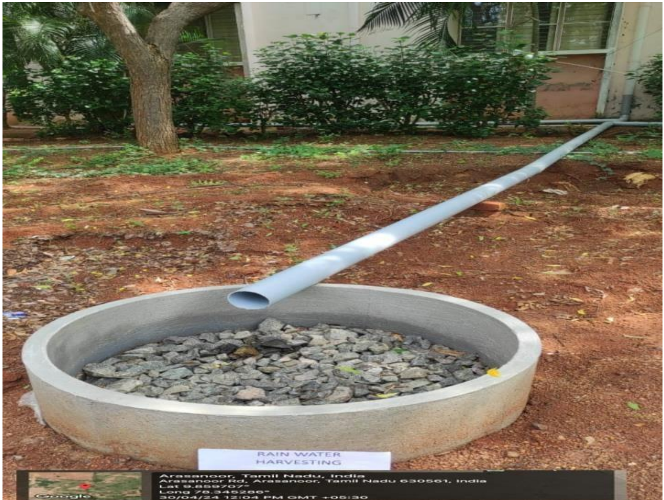
RAIN WATER HARVESTING
