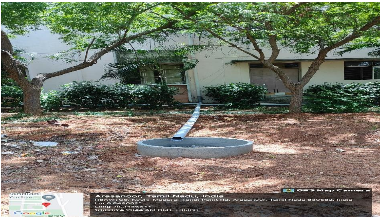
RAIN WATER HARVESTING
