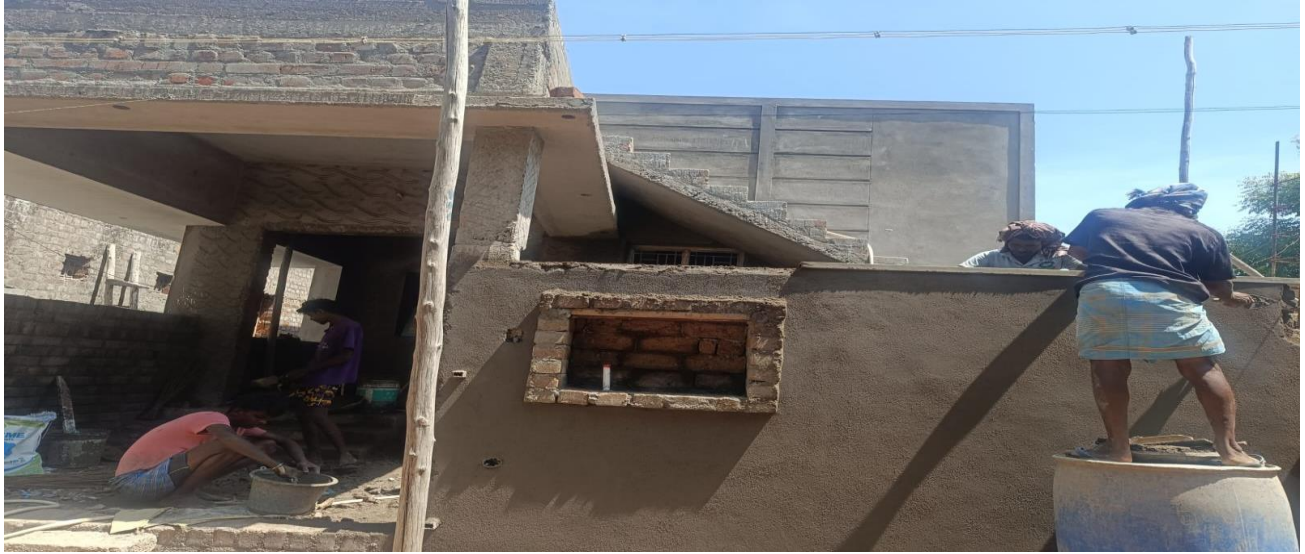
Best Engineers – Residential Building work at Idaya Melur Sivaganga – External Wall plastering
